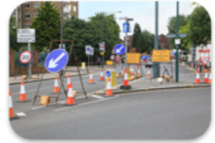
Traffic flow & speed is influenced by the road architecture
